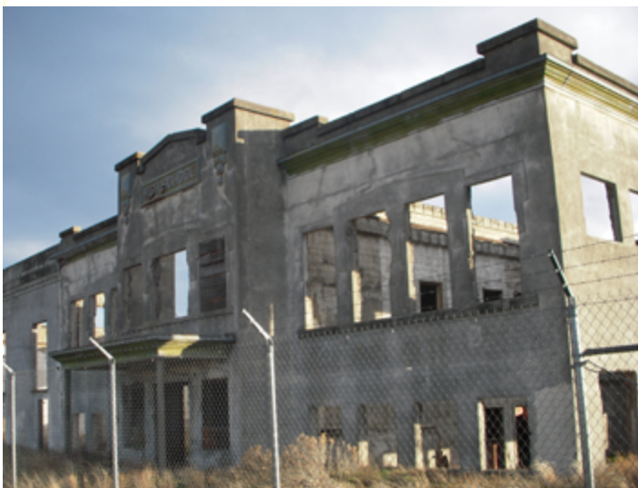
The historic Hanford high school
